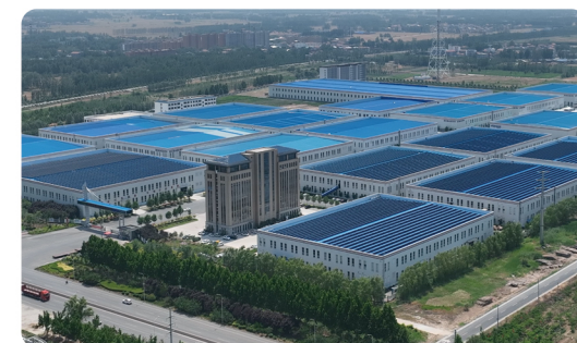
BIOBASE Juancheng County Medical Equipment Industrial Park
